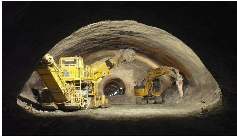
Tunnel Buchrain, Zubringer Rortal, Strassentunnel
